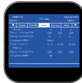
UPS Cabinet Control Panel
